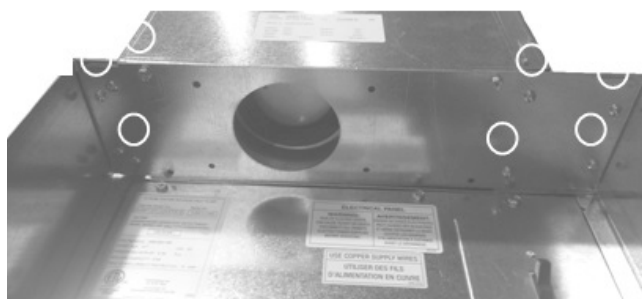
FIGURE 18 - STEP 1 - REMOVE DAMPER PLATE
