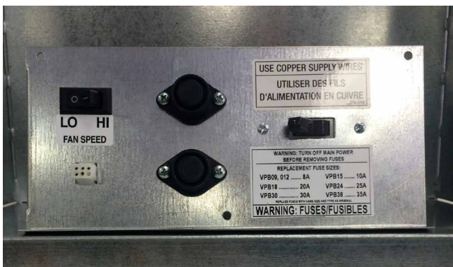
FIGURE 11 - UNIT SWITCH PLATE WITH ADA THERMOSTAT CONNECTION
