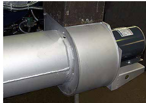
FIGURE 33 - FLUE COMBUSTION TEMPERATURE AND EFFICIENCY TEST PORT- ID BLOWER
