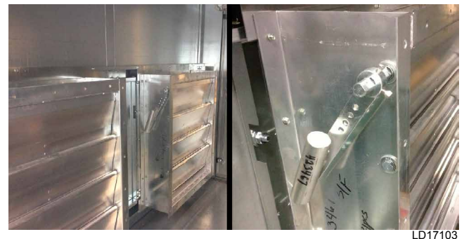
FIGURE 6 - COUNTERBALANCE LOCKED INTO PLACE FOR SHIPPING
