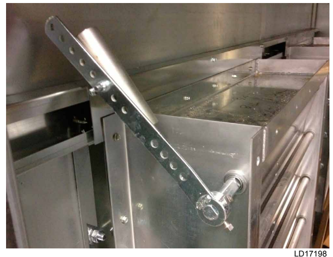
FIGURE 7 - COUNTERBALANCE UNLOCKED FOR START-UP
