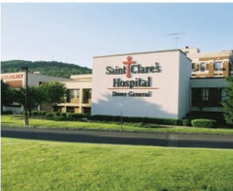
Saint Clare's Hospital - Dover General.
