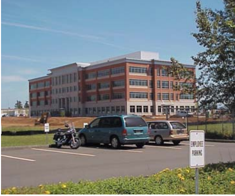
The PSB project is the first in a series of buildings that will house the county's operations in the coming years.
