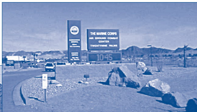
Under a comprehensive facility systems project, Johnson Controls upgraded five chiller plants on the base and installed a $16 million, 7 MW dual-fueled cogeneration system.
