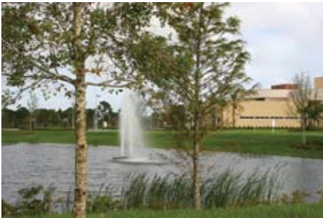
Holding ponds trap rain water for use in irrigation.
