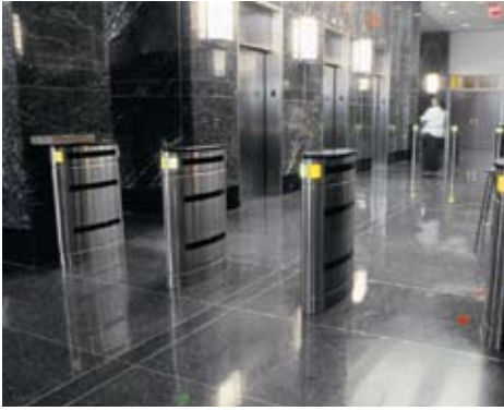
Electronic turnstiles are used at select facilities.
