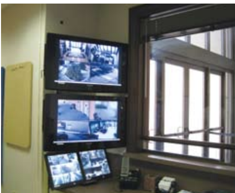
Security Control Room at the First Circuit Court of Appeal
