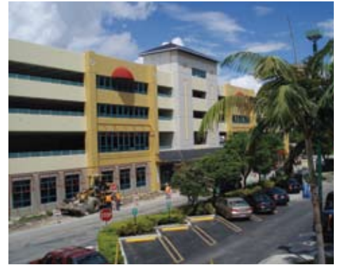
IP based video surveillance cameras allow security personnel to view intrusion points, campus-wide.
