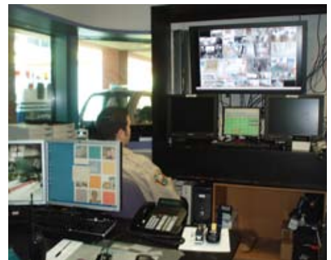
The new Central Operations Center will replace multiple dispatch stations.
