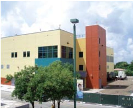
The new Central Energy Plant.
