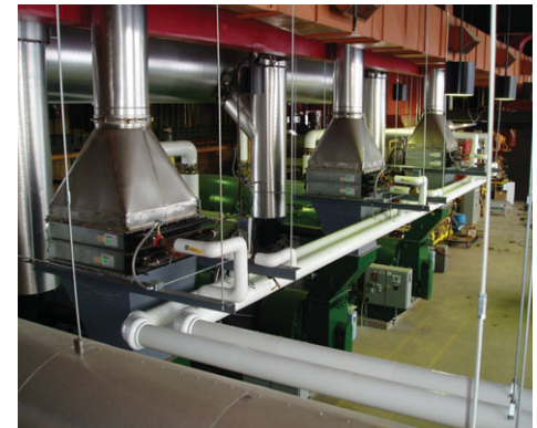
FRP pipe dramatically reduced installation problems.
