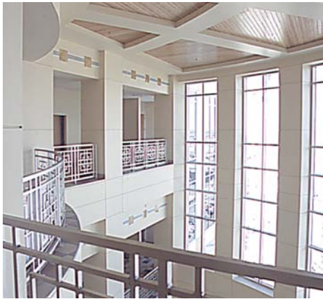
Ample daylighting provides a pleasing interior environment.
