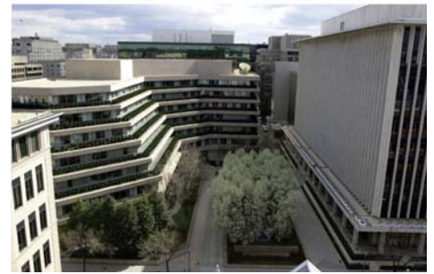
M Street building
