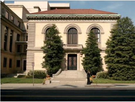
Hubbard Street building
