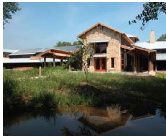
Schlitz Audubon Nature Center, Milwaukee, Wisconsin uses geothermal wells for heating and cooling
