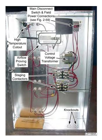
FIG. 2-58 – TYPICAL ELECTRIC HEAT CONTROL PANEL INTERIOR WIRING AND COMPONENTS
