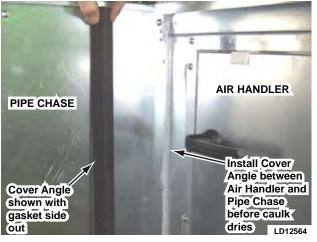
FIG. 2-48 - INSTALL COVER ANGLE
