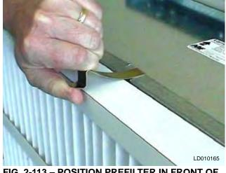
FIG. 2-113 – POSITION PREFILTER IN FRONT OF THE FINAL FILTER. (2" W/026-36339-000 LATCH SHOWN)
