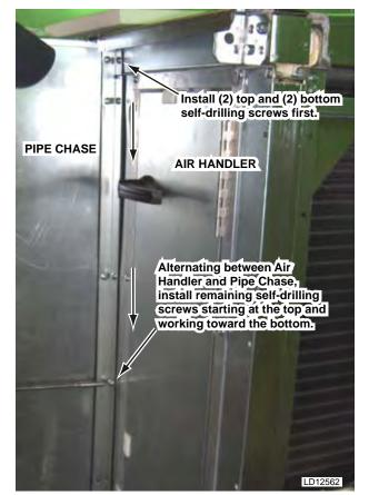
FIG. 2-50 – PROPER PATTERN FOR INSTALLING SELF-DRILLING SCREWS TO COVER ANGLE
