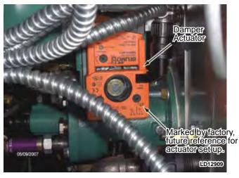
FIG. 3-19 – DAMPER ACTUATOR
