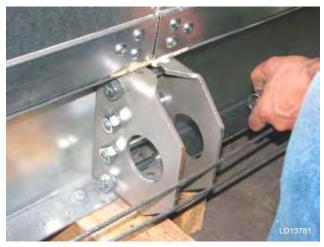
Use come-a-longs to pull the sections together. The bolts are to hold the sections tight after they are pulled together.
