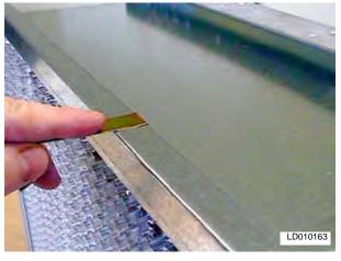
FIG. 2-112 – PREFILTER LATCH AFTER INSTALLATION ONTO FILTER HEADER.
