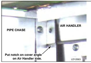
FIG. 2-49 – PROPER POSITIONING OF COVER ANGLE WITH NOTCH ON AIR HANDLER SIDE
