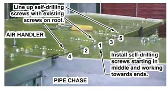
FIG. 2-46 – PIPE CHASE TO ROOF INSTALLATION
