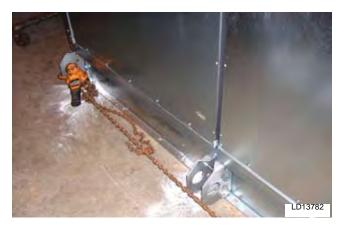
FIG. 2-25 – PLACING AND ANCHORING FIRST SECTION AND ATTACHING COME-A-LONGS
