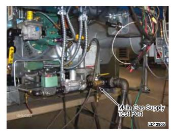
FIG. 3-16 – CHECK MAIN GAS SUPPLY PRESSURE
