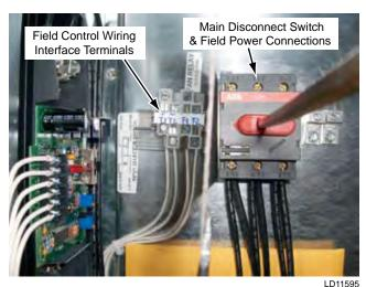
FIG. 2-59 – TYPICAL FIELD CONTROL AND POWER CONNECTIONS
