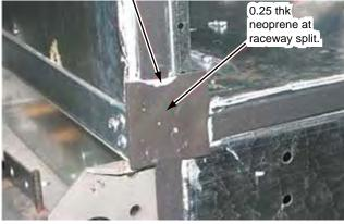
The gasket application should provide a continuous seal from side to side and the top of the unit roof to the bottom of the unit base where it meets the curb. LD13372A
