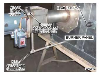
FIG. 3-15 – SET ID FAN DAMPER
