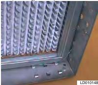
FIG. 2-103 - INSTALLED CARTRIDGE FILTER
