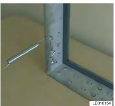
FIG. 2-107 – CORRECT LATCH/KNOCKOUT CONFIGURATION.
