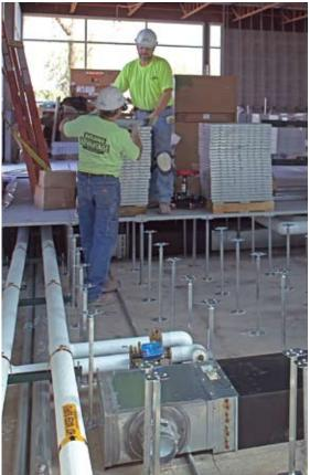
The FlexSys design provides easy access for utility service infrastructure and cabling during and after construction.
