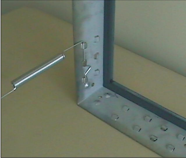
Figure 44 – Correct latch/knockout configuration.
