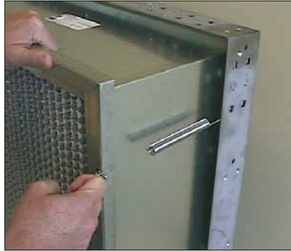
Figure 46 – Spring latch should be pulled and fastened in hole in the header of the filter.
