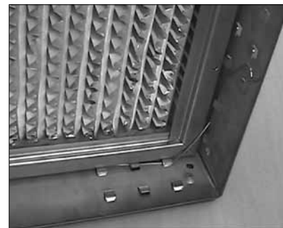
Figure 42 – Fully installed filter
