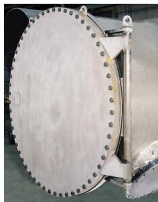
For easy tube cleaning, hinged water-box covers are available for the Titan chiller.
