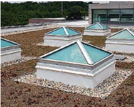
About 12,000 square feet of green roof absorbs precipitation, which reduces runoff, insulates the building, and extends the life of the roof. Skylights reduce the need for lighting inside the buildings.
