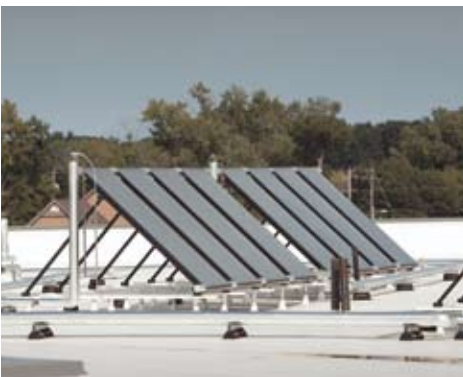
Solar thermal systems supply more than 30 percent of the hot water needs for two buildings.
