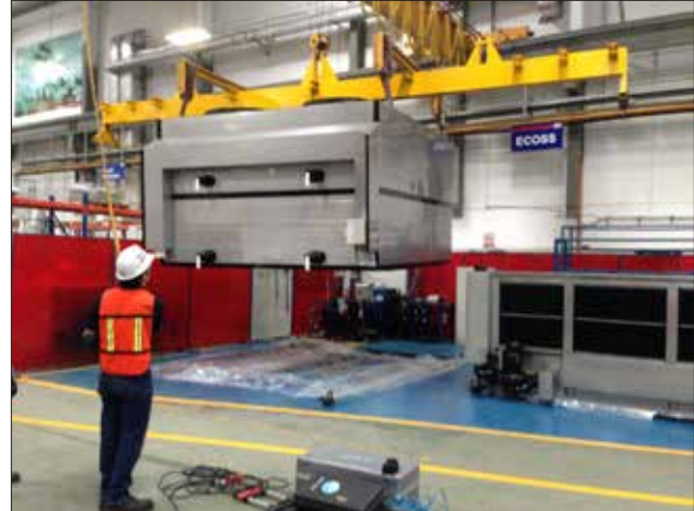
Figure 12 - Lifting Top Section of the Unit
