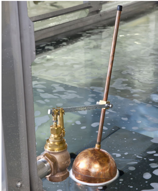
Figure 4. Mechanical Float Valve
