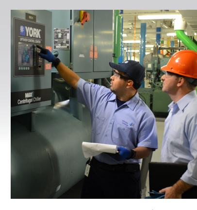
extremely leak tight. Similarly, so do low-pressure (R11, R123) centrifugal chillers, so it's critical to check for leaks and maintain the purge unit components to ensure reliable operation and long equipment life. Over the past 10–15 years, variable speed drives have become prevalent on centrifugal chillers. These drive and control components are complex and, as discussed earlier, are best addressed during seasonal start-up by highly trained technicians, such as those trained by OEMs.
