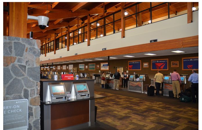
Axis PTZ cameras placed throughout the airport monitor the ticketing/check-in area.
